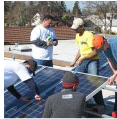
Volunteers performing a tilt-up solar installation in Pleasanton in February.
