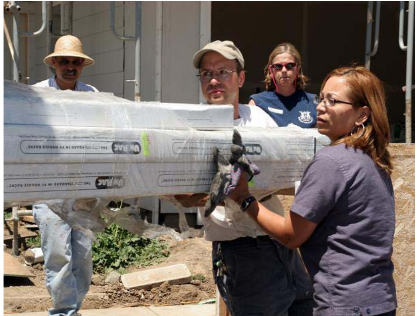
Our wonderful volunteers carrying rails for the solar installation in Livermore. The nine systems range from 1.1kW to 1.6kW in size, reducing annual electricity costs by $300.
