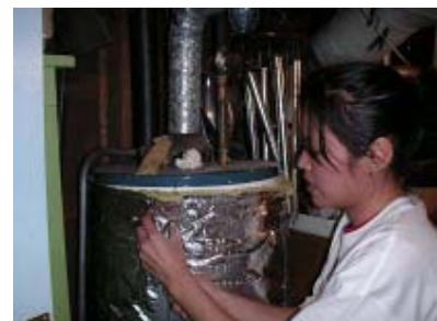
A volunteer installs a water heater blanket in San Francisco for the Energy Efficiency Team with Rebuilding Together. Measures like these will help reduce the cost of utilities by $189 per year for low and fixed-income seniors
