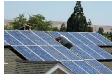
On June 4th and 5th, volunteers from GRID Alternatives and East Bay Habitat for Humanity installed solar panels in Livermore for habitat’s development. Over 100 volunteers participated in the project.
